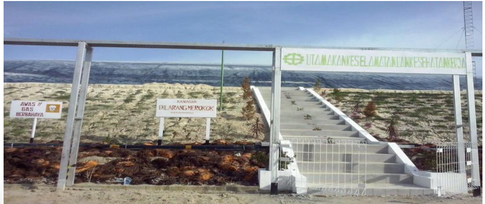
Biogas POME Power Plant in Rokan Hulu, RIAU Biogas : 750 m 3 /hour (60% CH 4 ) Utilization : 1 MW for 1 050 household
